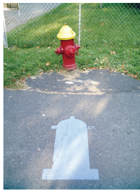
Road markers painted on road in front of hydrant.
