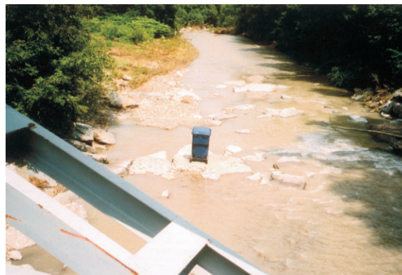
Trash can in Keshequa Creek near wastewater plant site.
