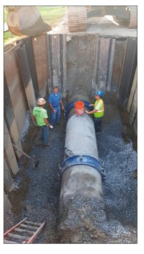
a long-term repair solution. They can absorb post-installation dynamic pipe deflection of up to 4° on each end to absorb pressure on the pipe due to shifting ground and changing temperatures. The deflection helped reduce the risk of damage and cracking while saving resources on constant future pipe repairs.
