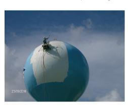
In spections should also include but not be limited to ultrasonic testing, which detects the thickness of steel; dry fill thickness tests determine how thick the paint is, and crosshatch tests measure
