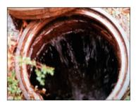
manholes can contribute significant inflow and infiltration through leaky covers. 3D manhole scanning technology can inspect manholes and uncover these defects. If a manhole inspection reveals I & I there are a few repairs available to quickly reduce inflow. Including replacement of manhole covers, sealing covers and resetting cover rings, chemical grouting to seal up leaking joints and epoxy lining of the manhole.
