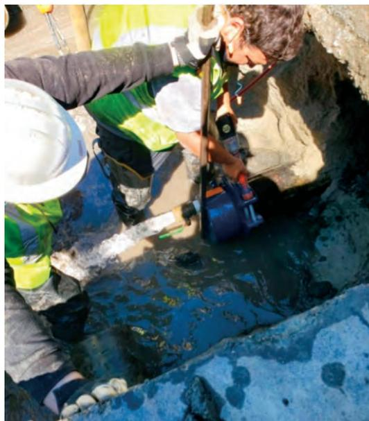
The HYMAX GRIP has a universal gripping system designed to restrain metal and plastic pipes and has a transition capability of up to 1.1". It can work with a wide range of pipe diameters, meaning that John had extra flexibility to use the GRIP for a variety of other pipe sizes he might find in the ground.
