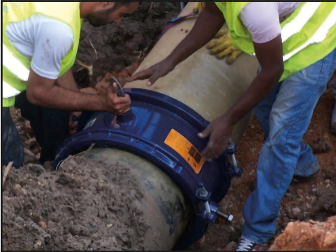
HYMAX coupling being installed. Be sure to keep your inventory stocked with at least two repair products on the shelf for each to minimize time handling emergencies.
